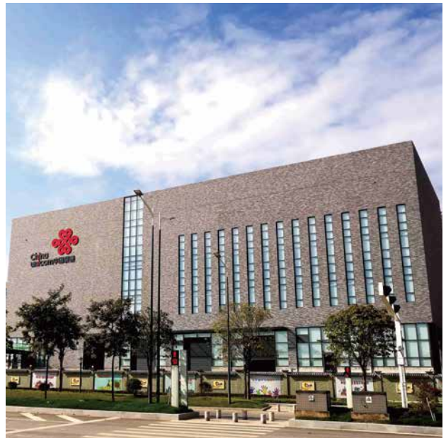
China Unicom Cloud Data Center Project
