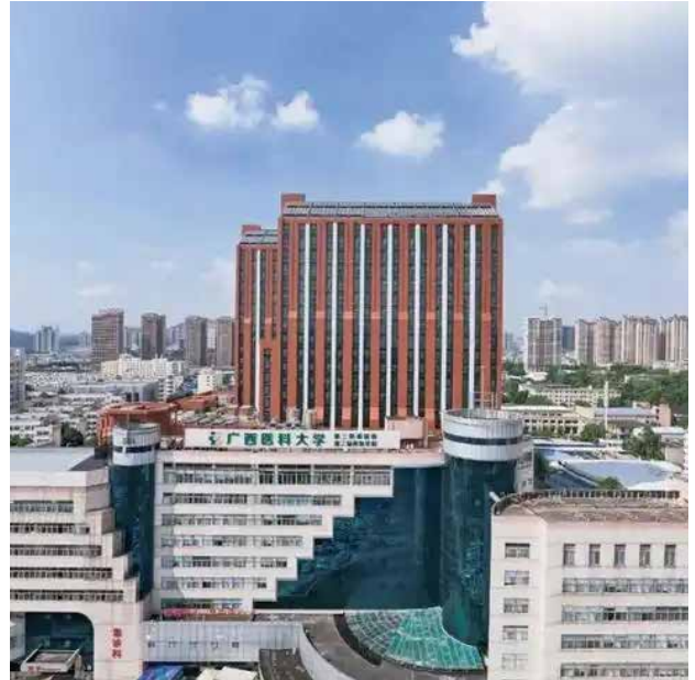
Guangxi Medical University Second Affiliated Hospital Project
